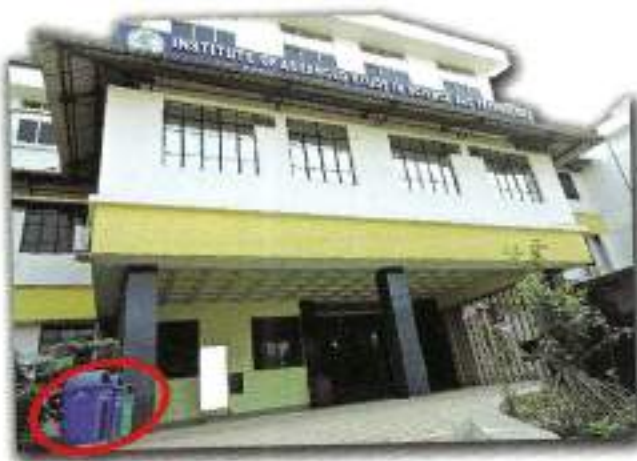
Fig1: Dustbins in front of main Entrance Gate
